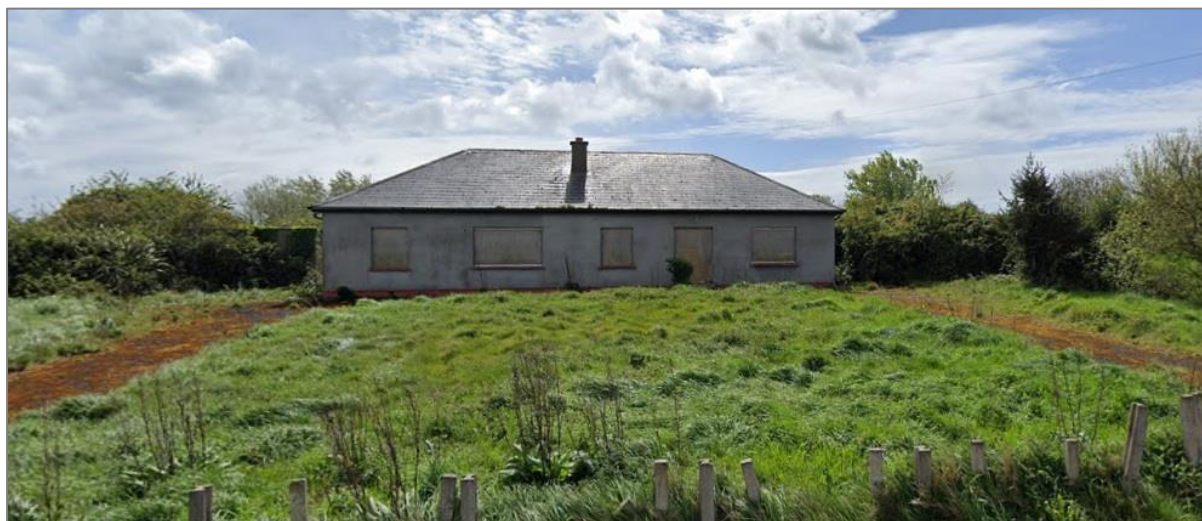
Figure 13.10 Bungalow to be demolished
