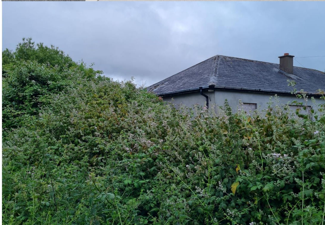
Plate 6. New road. Plate 7. Derelict house
